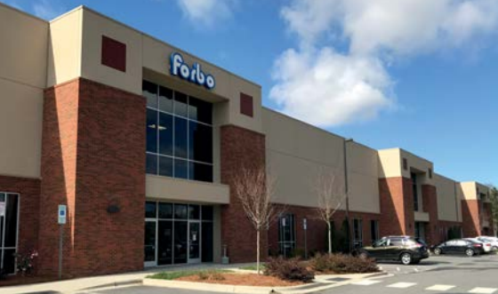
◀ FORBO Production and Distribution Center Huntersville, North Carolina (Charlotte MSA)
