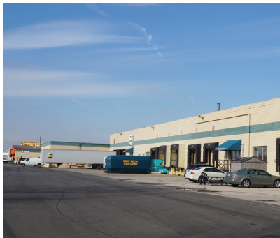
Interline Brands (Home Depot subsidiary) Industrial Distribution Center Louisville, KY
